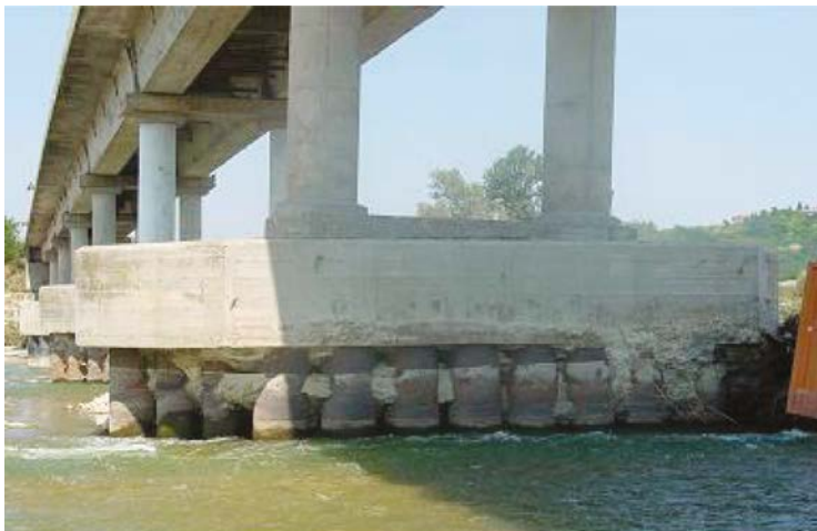
Figure 2.20: Bed degradation of the Tanaro River (Piedmont, Italy) at Barbaresco-Molini d'Isola d'Asti has given rise to the severe erosion of the bridge piers (Seminara et al. (2003)).
