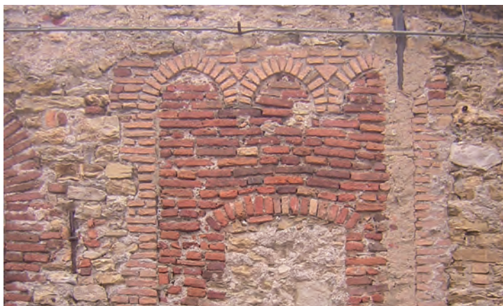
Fig. 15 - Stratification of the walls with the possibility of mensiochronological dating
