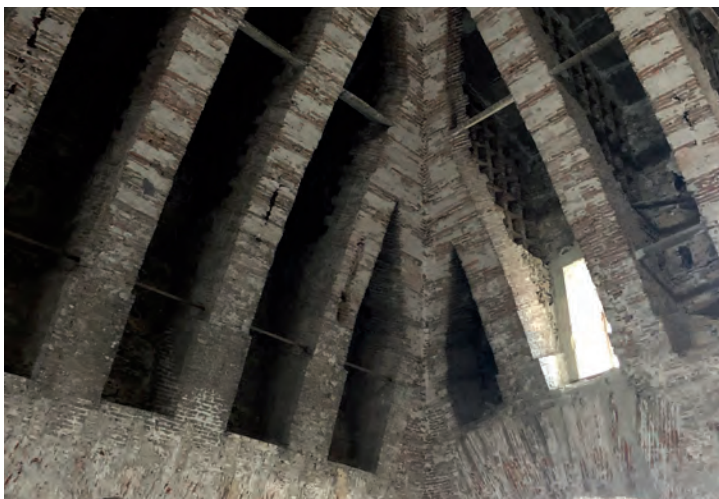
Fig. 22 - View of the structural ribbed vault in the roof masonry above the Sala del Minor Consiglio
