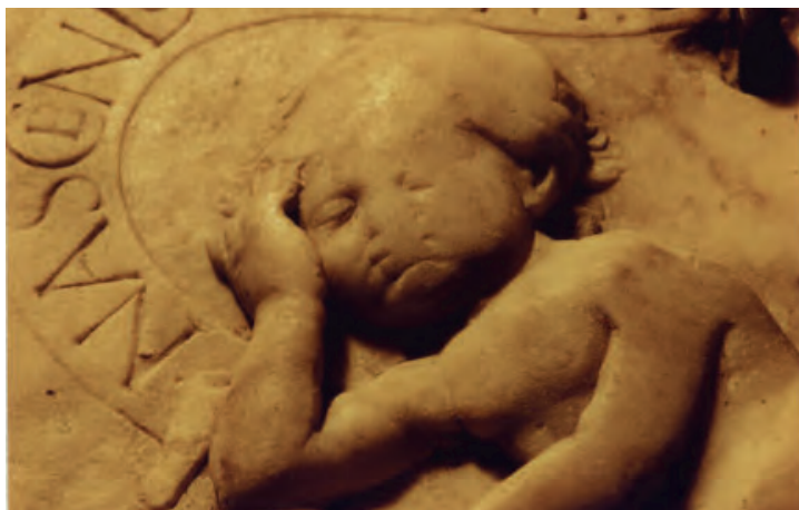
Fig. 262 - Signs of degradation on a marble tomb. The phenomenon can be defined as erosion, according to the Lexicon of Recommendations UNI 11182
