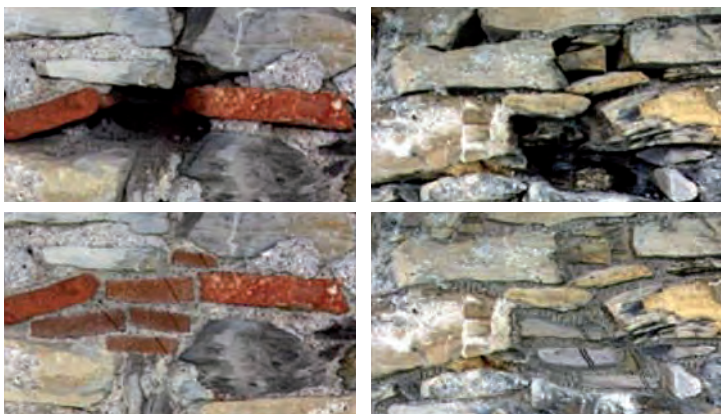
Fig. 258 - Simulation of an operation to integrate the building material by inserting stone material and grouting the joints
