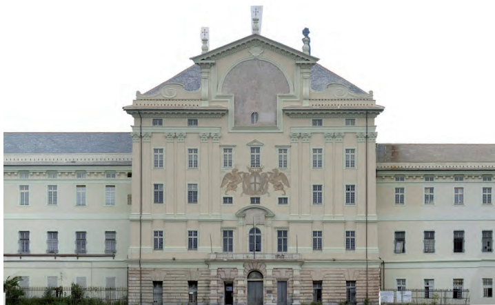
Fig. 39 - Reinstatement of the photogrammetric survey of the south facade of the Albergo dei Poveri: partial view of the orto-photo of the main front
