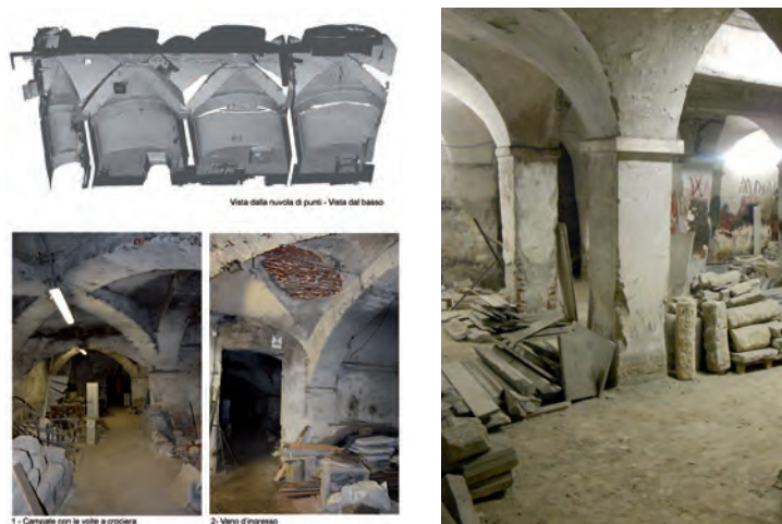
Fig. 32 - Digital relief of the ribbed vaults on the lower floors of the Villa del Principe Doria: views of the point cloud and of the rooms on the lower floors
