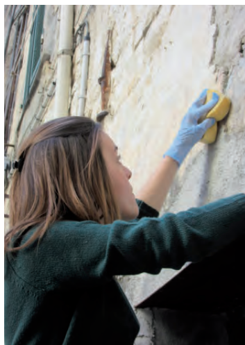
Fig. 57 - Treating the edges of an area without plaster
