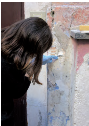
Fig. 58 - Plastering with compatible mortar
