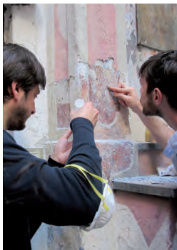
Fig. 59 - Removing lime using a scalpel and re-adhesion with injections
