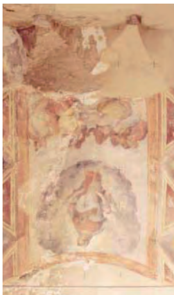
Fig. 215 - View of the internal vault in an advanced state of disrepair, mainly due to water infiltration
