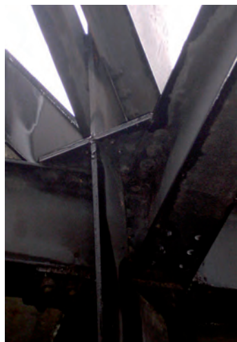
Fig. 160 - Detail of the interlocking elements on the edges of the outer framework
