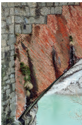
Fig. 226 - Examples of alterations and degradation: overgrown vegetation and carbonate deposits
