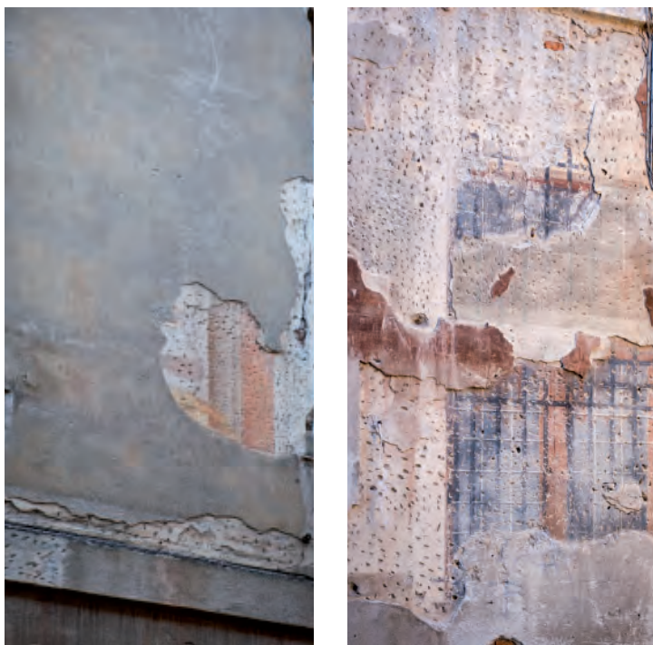
Fig. 200 - Details of the facade on via Roma. To the left, detail of a missing layer of more recent plaster. To the right, detail of the decoration of the facade visible through the missing parts
