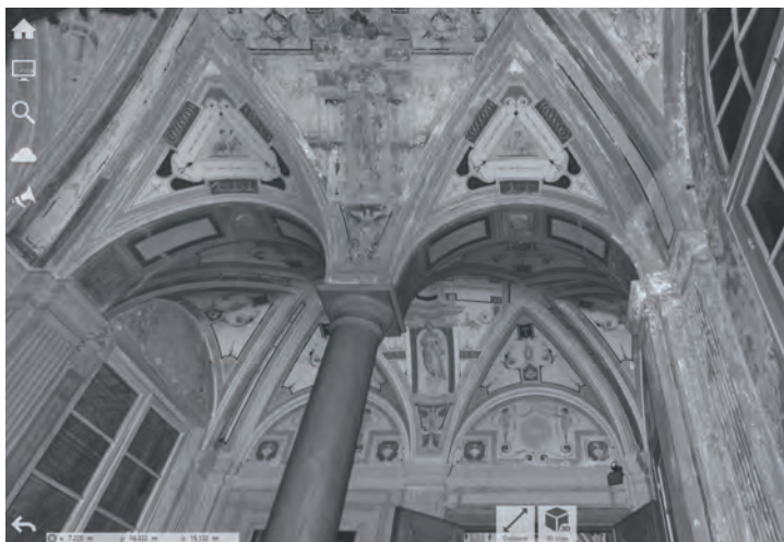
Fig. 8 - View of the point cloud obtained by laser scanner survey. Vault of the loggia of the “piano nobile” (main floor) of Palazzo Belimbau, Genoa
