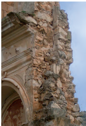
Fig. 190 - Detail of the cross section of the perimeter wall of the church
