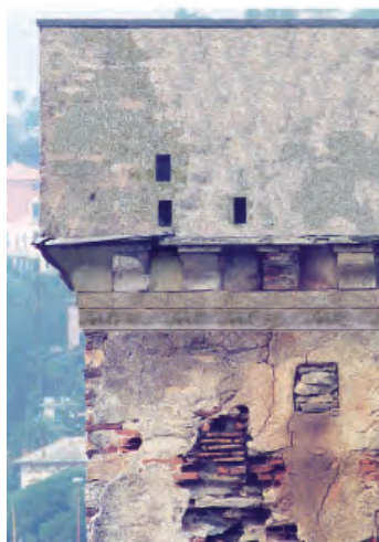
Fig. 272 - Simulation of an operation of consolidation using cerclage with a carbon strip later plastered
