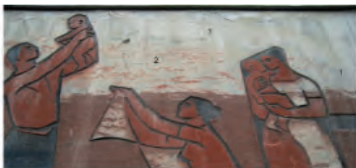
Fig. 131 - Detail of the degradation of the graffiti of Janos Blaski: interruptions in the continuity of the graffiti owing to cracks
