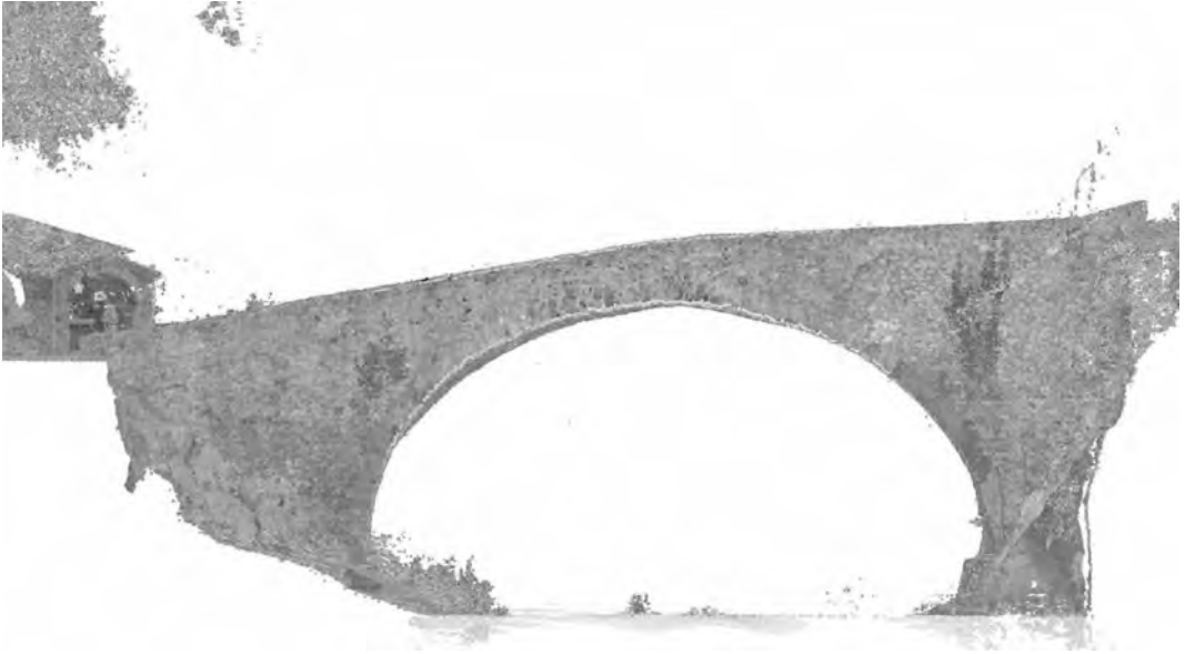
Fig.5 Prospectus of the Bridge of San Michele obtained from the Union of the point cloud
