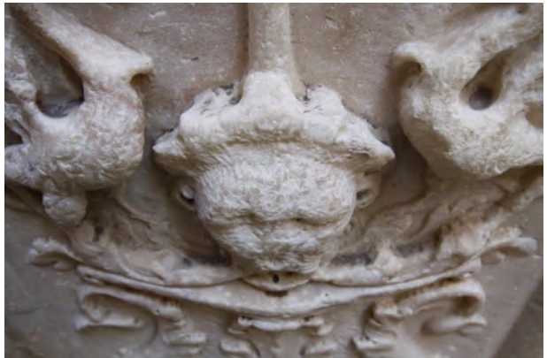
Fig.14 - Dissolution of calcareous stone surfaces exposed to water runoff
