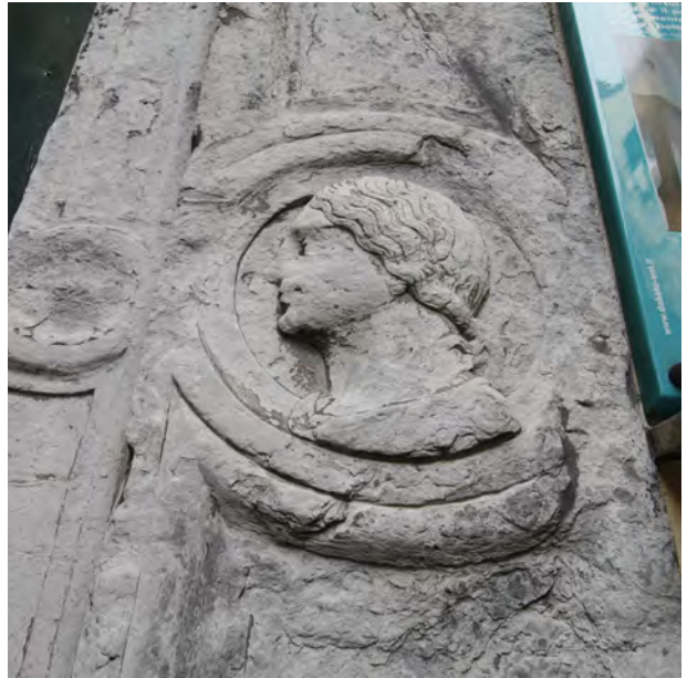
Fig.10 - Dissolution of calcareous stone surfaces exposed to water runoff
