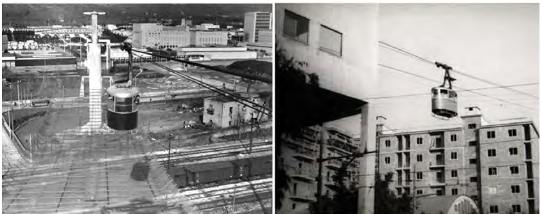
Fig.2 The ropeway, seen from the hill towards the valley (left), and near Viale Kennedy, from the Cumana railway (right).
