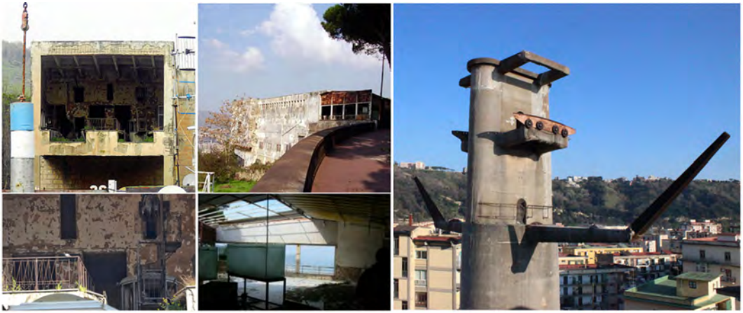
Fig. 5 A series of images of the abandoned ropeway. Top left, the two stations, lower and upper; with the equipment and an old cabin; below, exterior and interior of the upper station. Right, the upper part of one of the impressive pylons.
