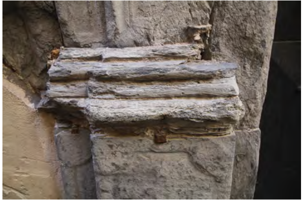
Fig.12 - Exfoliation: detachment of multiple thin stone layers (cm scale) that are sub-parallel to the stone surface.
