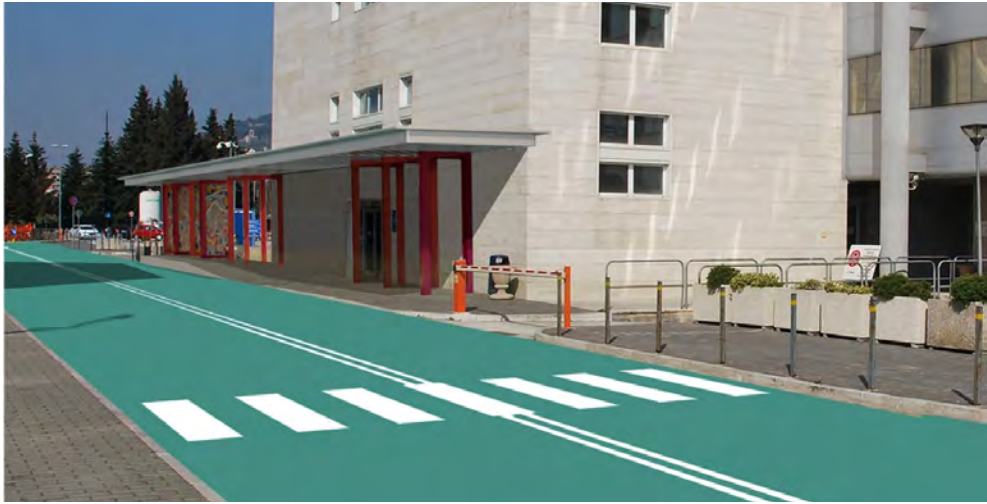
Fig. 2 The high solar reflection coating of the path on the BRT's premises by the University stop.
