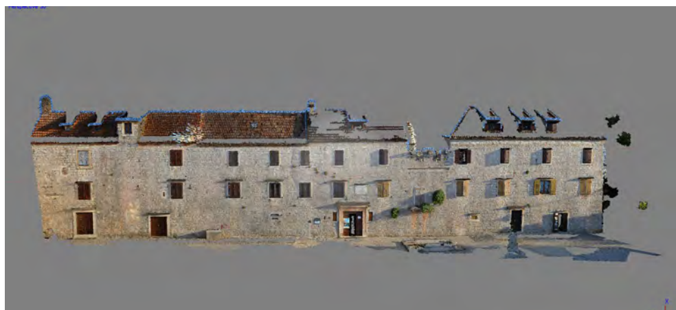
Fig. 1 The Fortress of Hvar Tvrđalj, cloud of points on the outer elevation overlooking the main square
