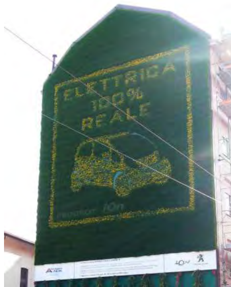
Fig. 1 Temporary installation of a vertical greening system in Milan (Italy)
