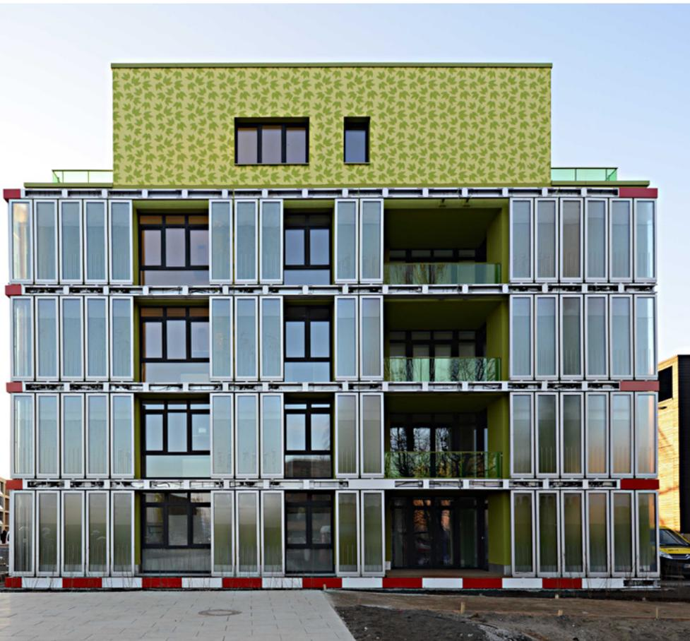
Fig. 1 Bio-adaptive façade of the BIQ House, by Splitterwerk Architects + Arup group, Hamburg, 2013 <https://www.arup.com/projects/solar-leaf>
